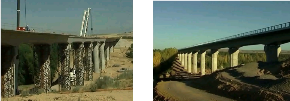
Figure 11: Río Moros viaduct (Courtesy of PRAINSA).
