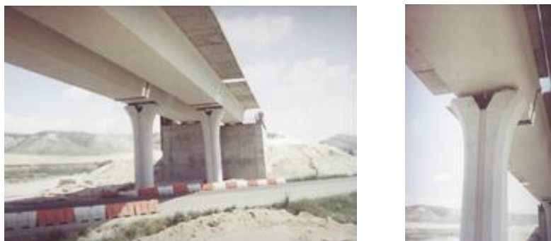
Figure 12: Double box section bridge (Courtesy of PRAINSA).
