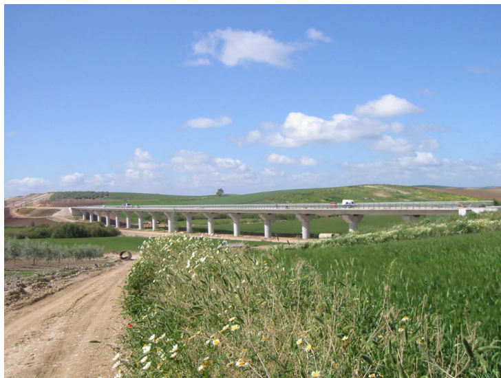
Figure 6: Río Cabra viaduct (Courtesy of NECSO).
